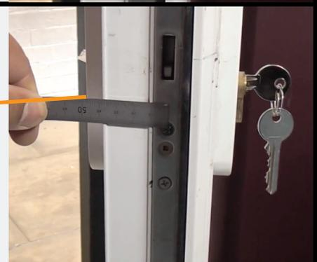
Replacing a Euro cylinder on the vast majority of doors is a simple process. The only tool required is a crosshead screwdriver.
